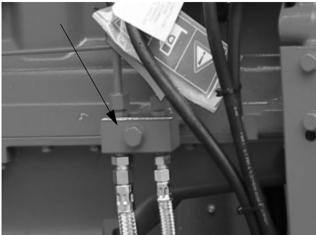
Fig. 22 Connecting the fuel pipes to the connecting block
